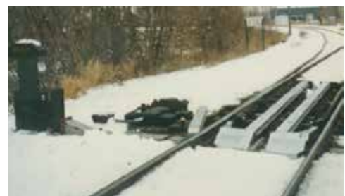
Railway switch heater Forced heated air directed through ductwork that melts snow and ice from switch components.
